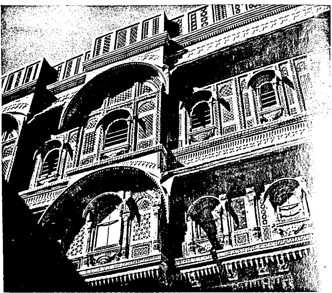
Carved and jali work windows and arches of a yellow-brown sandstone house in Jaipur, Rajasthan.
